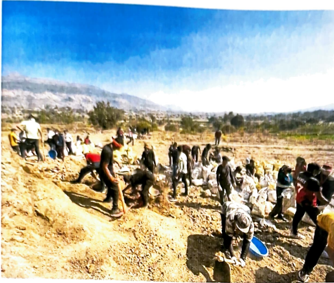
Photograph no.: -15 Excavation for Dam Construction
