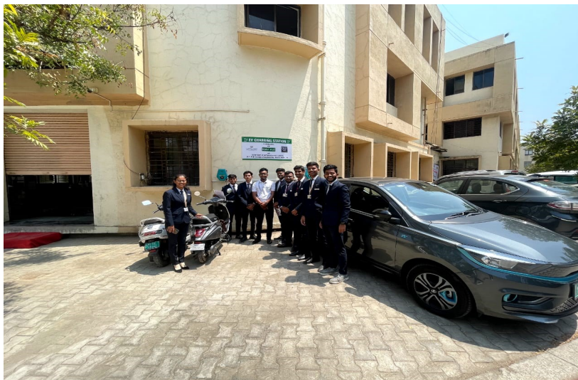
Testing of EV Charging Station by Experts of Virtuoso Projects and Engineers Pvt Ltd, Pune
